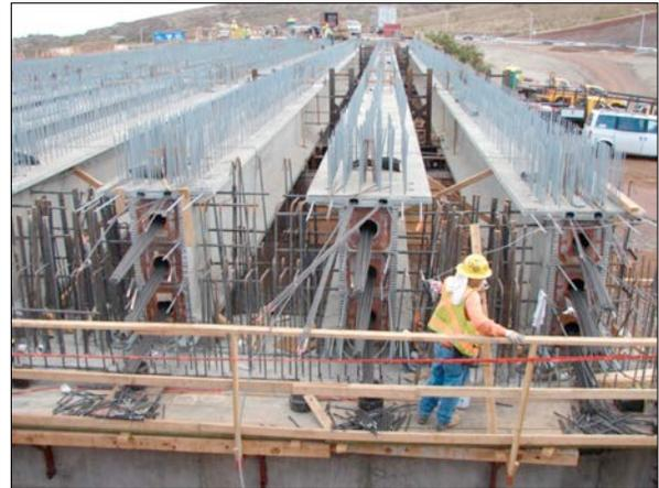
**Cortec's MCI®-309 Powder provides corrosion protection of metal tension cables without the need to drill multiple holes along the length of the members to be treated.**
