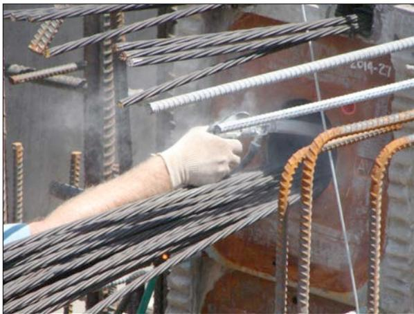
MCI®-309 is applied as an aerosol suspension (dry fogging) into the casing surrounding the metal element to prevent corrosion.
